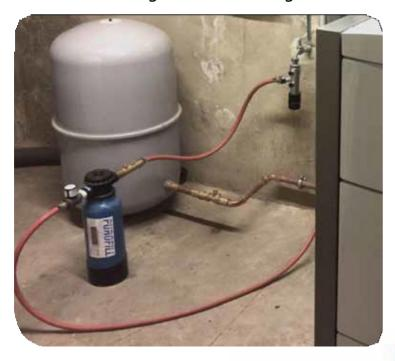
Filling heating systems with demineralised water is now a go to standard in order to maintain the systems in terms of performance and value.
